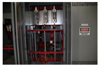
Service Entrance w/ metering compartment – 1200A, 31.5kA, 26.4kV, 150kV BIL (38kV Class)
