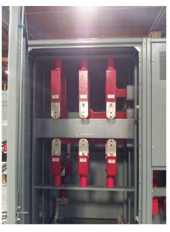
Service Entrance w/ EUSERC metering compartment - 1200A, 5kV, 25kA
