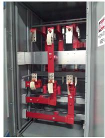
Outdoor (non-walkin) Service Entrance w/ EUSERC metering compartment – 1200A, 12kV, 25kA
