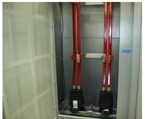
Outdoor (Non Walk-in) Service Entrance w/ metering compartment – 38kV, 600A, 31.5kA, 150kV BIL
