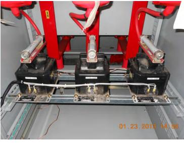
Service Entrance w/ metering Compartment – 1200A, 15kV, 25kA
