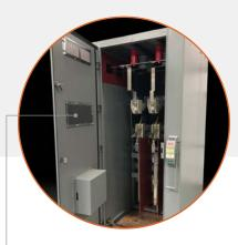
VIEWING WINDOW TO VIEW SWITCH POSITION FOR SAFETY
